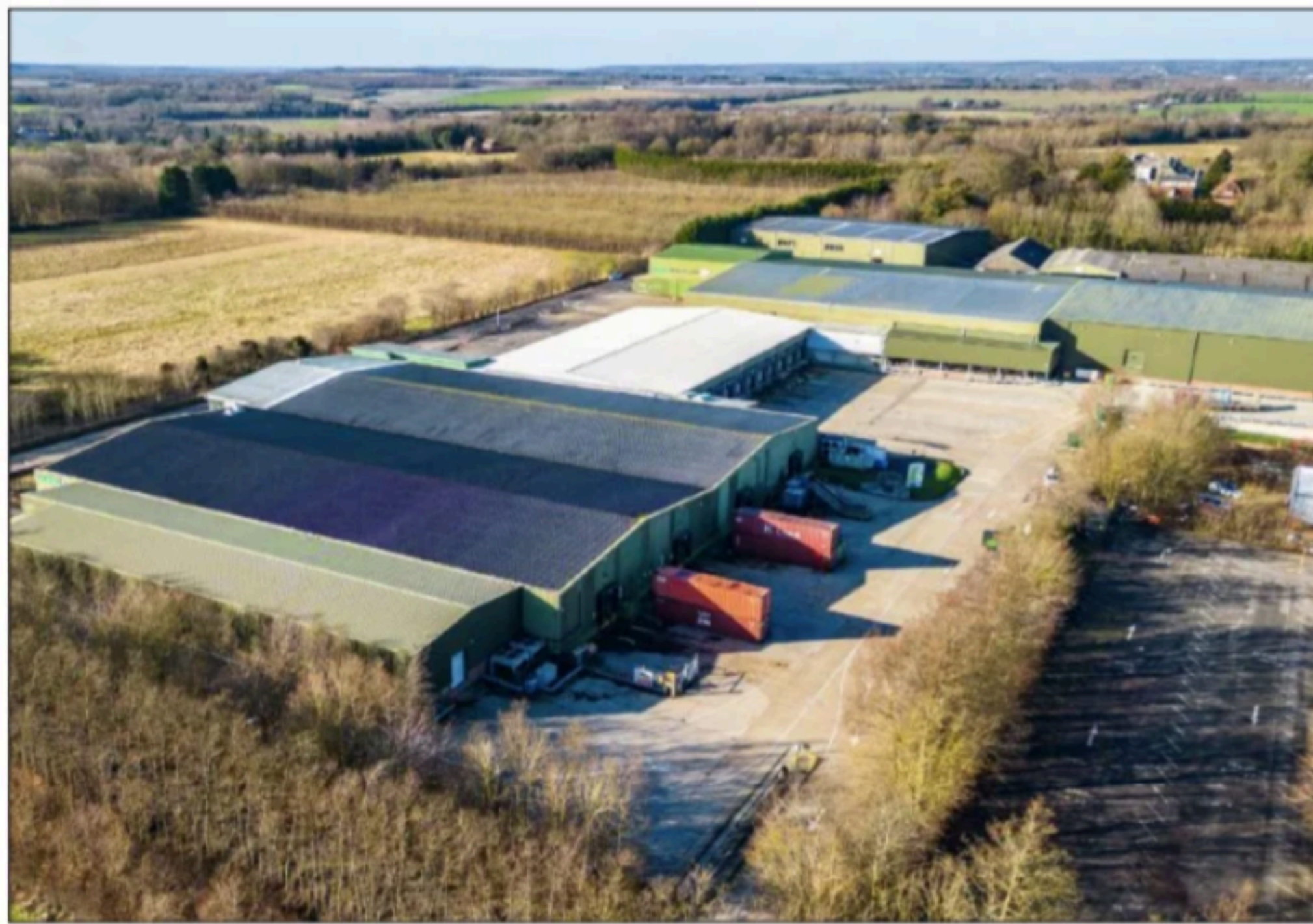
The sprawling 10.4-acre former A Gomez site in Bridge is up for sale
